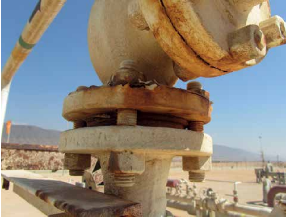
Above: Flanges damaged by corrosion
