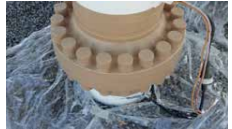
Above: Application of first coat of Belzona 3411
