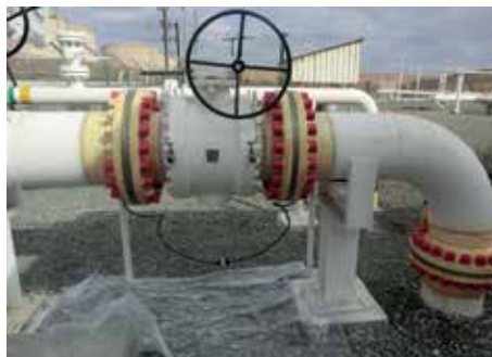
Above: Surface prepared, Belzona 8411 applied and bolt caps installed
