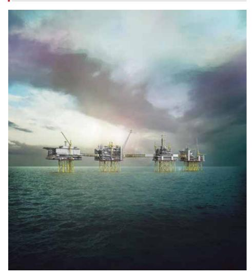
The Johan Sverdrup field is planned as a phased development, with a Field Centre and tie-backs of subsea templates and standalone well head platforms. The field is located on the Utsira Height in the North Sea, approximately 155 km west of Stavanger and near to the fields of Grane, Ivar Aasen, Edvard Grieg and Sleipner.
