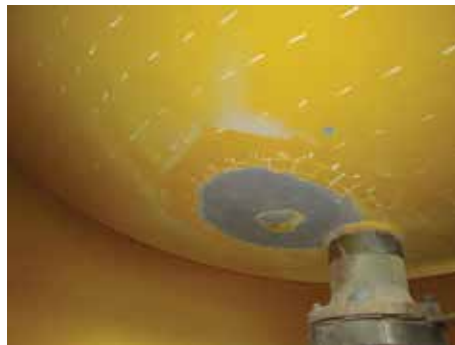
Above: Belzona 1212 heals thin and through-wall defects
